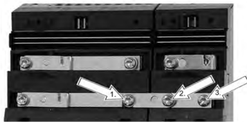
1. Connection of the lower DC link busbars
